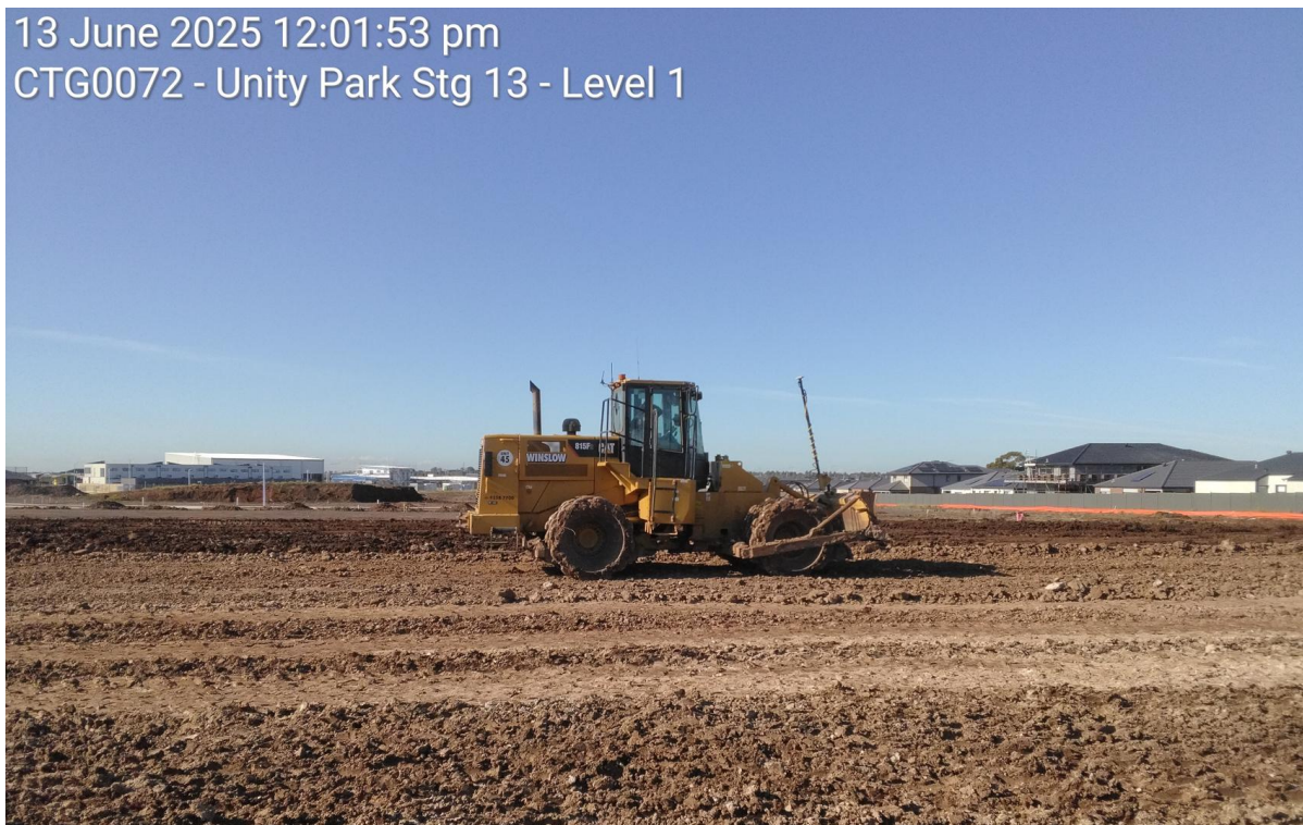
Figure 3: Fill Compaction (Source: C&T)
