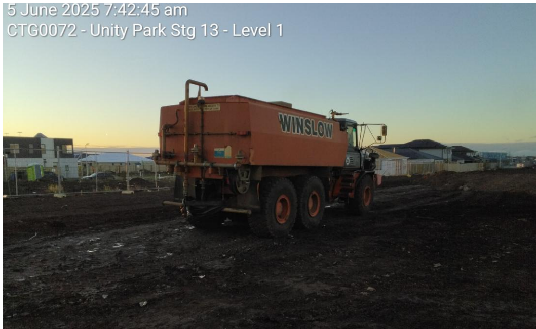
Figure 1: Subgrade Test Rolled & Moisture Conditioned (Source: C&T)
